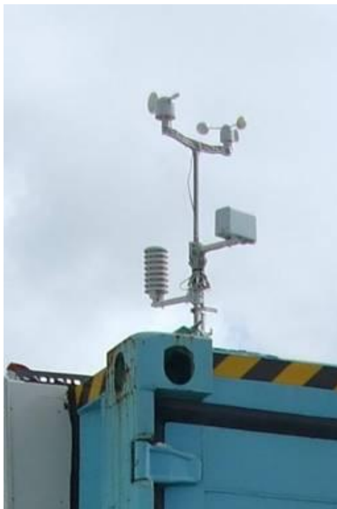
Figure 3.2: Weather sensors located on the container roof.
