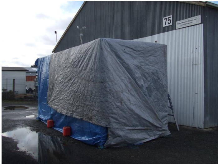
Figure 3.9: Tarpaulins used to cover the container.
