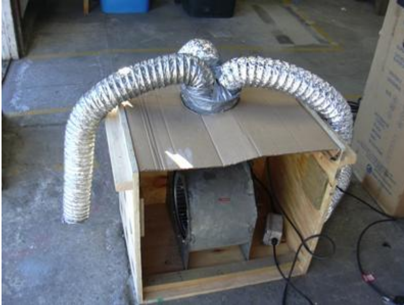
Fig. 3.11: The auxiliary fan fitted with three outlet hoses.
